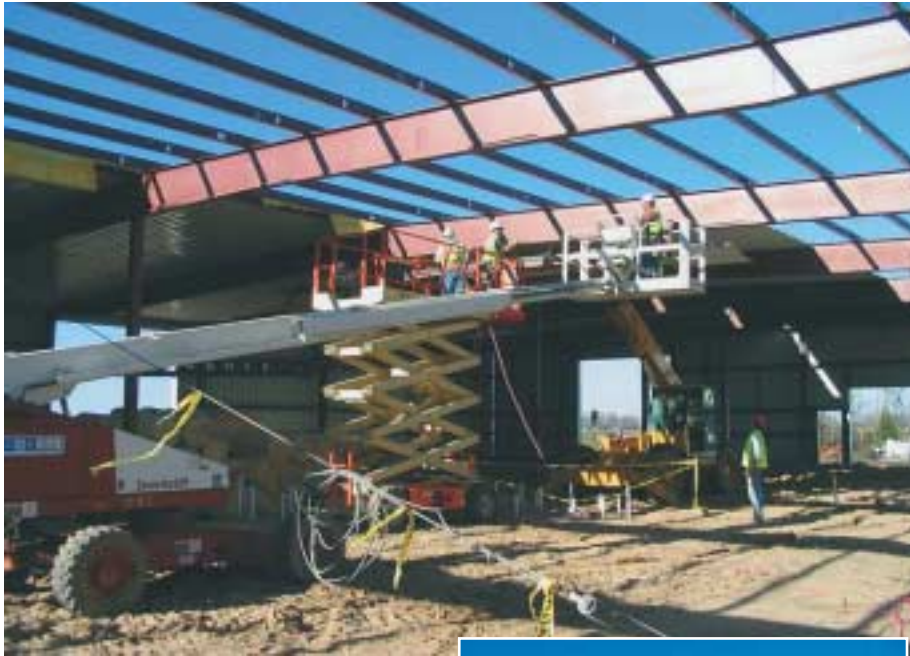
Constructing the metal building at Monsanto in Glyndon, Minn.
