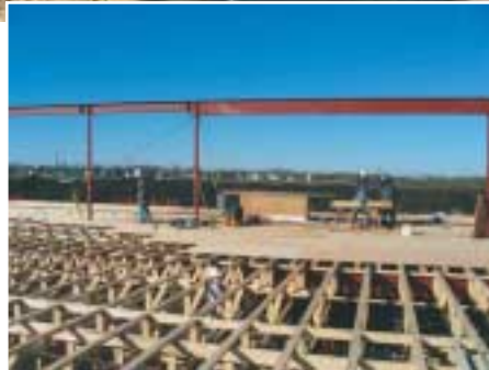
Crews setting floor trusses at Titan Machinery in Fargo, N.D.
