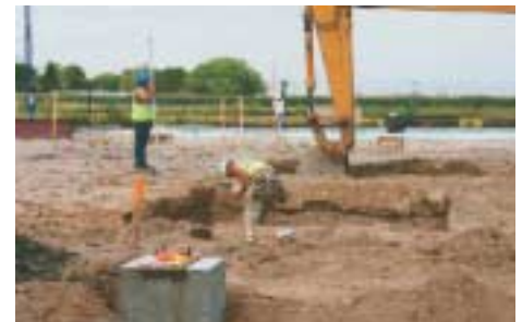
Pictured above left: Olaf Anderson & Son carpenters establishing the correct grade for pad footings. Above right: Olaf Anderson & Son Construction concrete crew members forming a center pad at the North Dakota State University Health and Wellness addition in Fargo.
