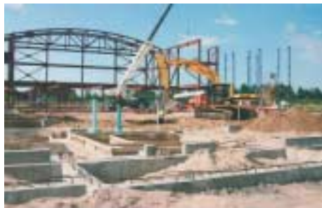
Pictured above left: Olaf Anderson & Son carpenters establishing the correct grade for pad footings. Above right: Olaf Anderson & Son Construction concrete crew members forming a center pad at the North Dakota State University Health and Wellness addition in Fargo.
