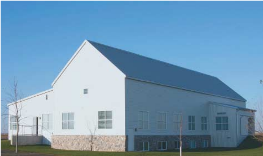
Real fieldstone, galvanized and corrugated roofing and large windows are just a few of the common design elements seen throughout Rocking Horse Farm.
