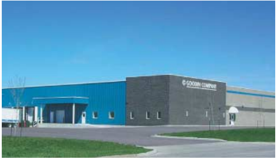
An exterior view of the Goodin Company in Sioux Falls, S.D.
