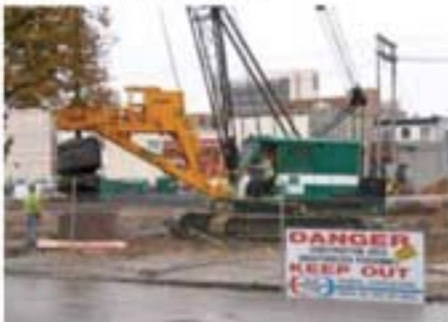
Caissons being drilled to a depth of 107 feet and filled with concrete.
