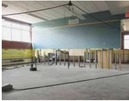
Above left: Olaf crews survey the damage in the basement of Benson Hall. Center: Water damaged classroom walls were removed to four feet to prevent mold. Right: Flood damage to the Home Economics classroom.
