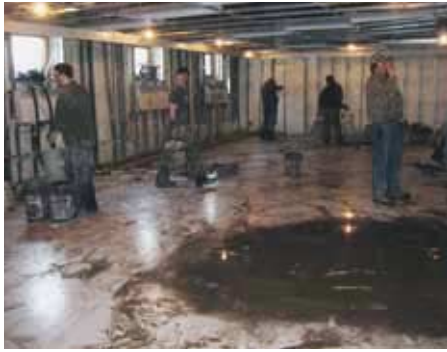
Above left: Olaf crews survey the damage in the basement of Benson Hall. Center: Water damaged classroom walls were removed to four feet to prevent mold. Right: Flood damage to the Home Economics classroom.
