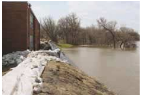
One week after the crest, the water is no longer at the top of the dikes, but the football field on the right remains under water.
